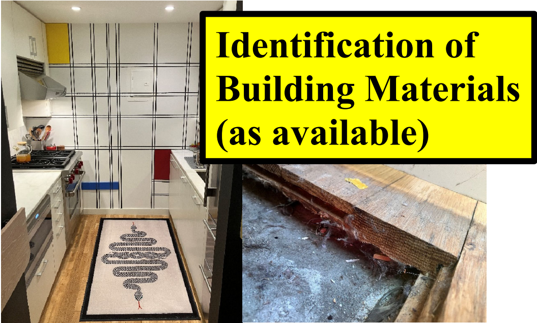
> A “floating” solid tongue & groove wood floor was installed in kitchen/hallway/living room/bedroom.
