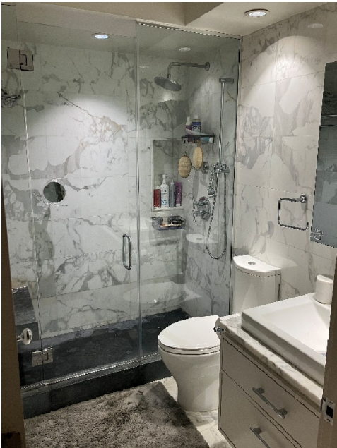
> Marble floor tile appeared to be installed in the bathroom.
